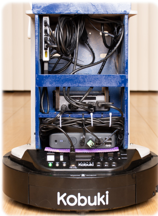
Figure 10. The inside of the lower base where the battery, computer, and wiring are housed.
